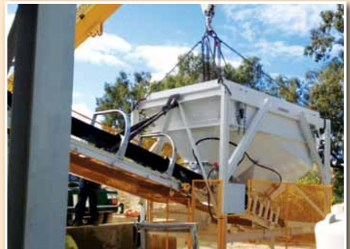
This picture shows a new weigh hopper and conveyor being installed at Rochester.
